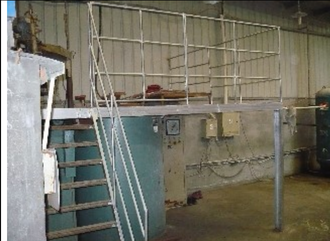
Handrails for ladders and guardrail for platform
